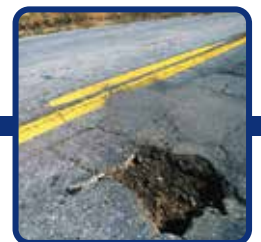
POTHOLE/DAMAGED PAVEMENT
